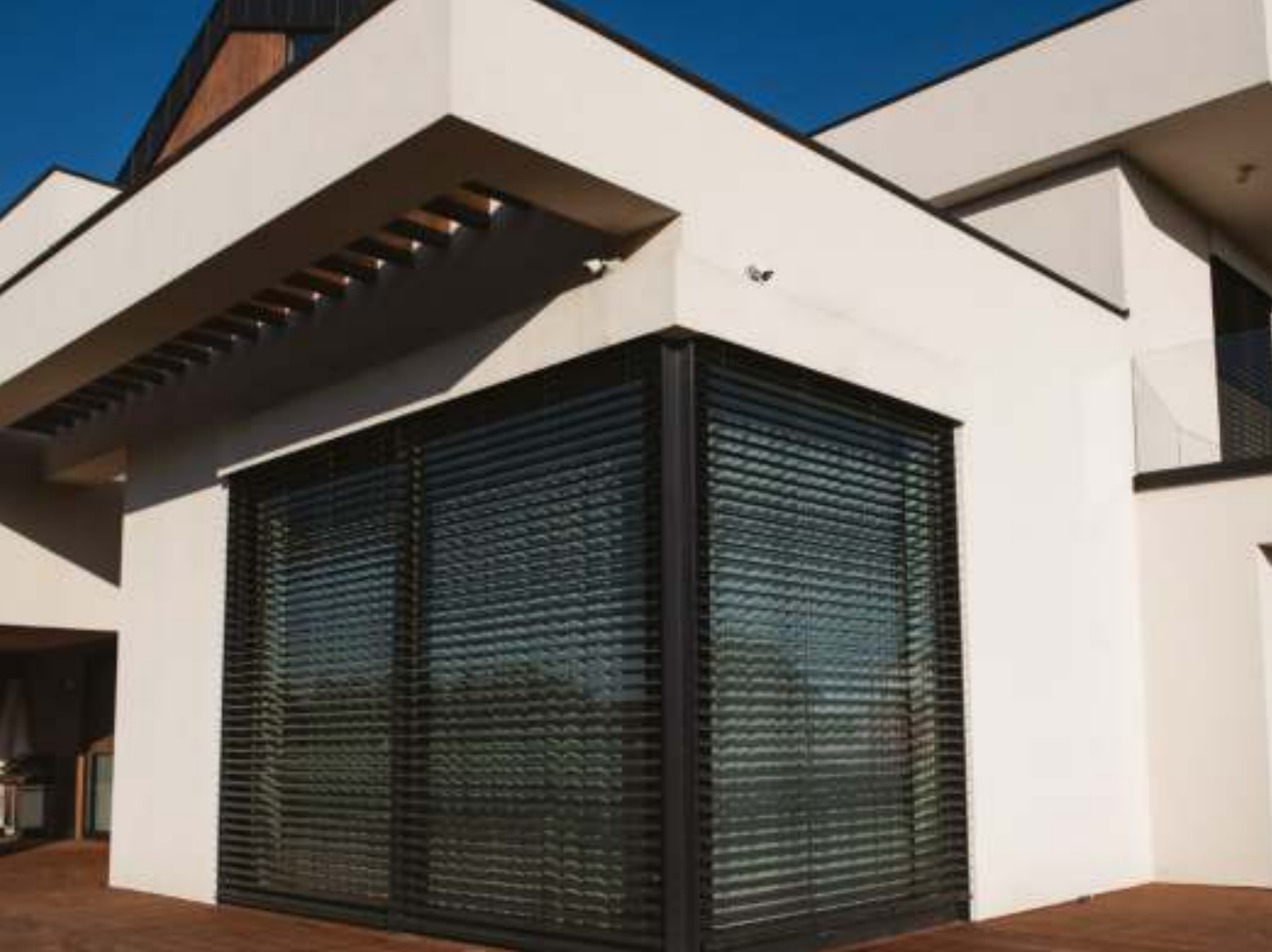
Flush-mounted façade shutters, Single-family house
