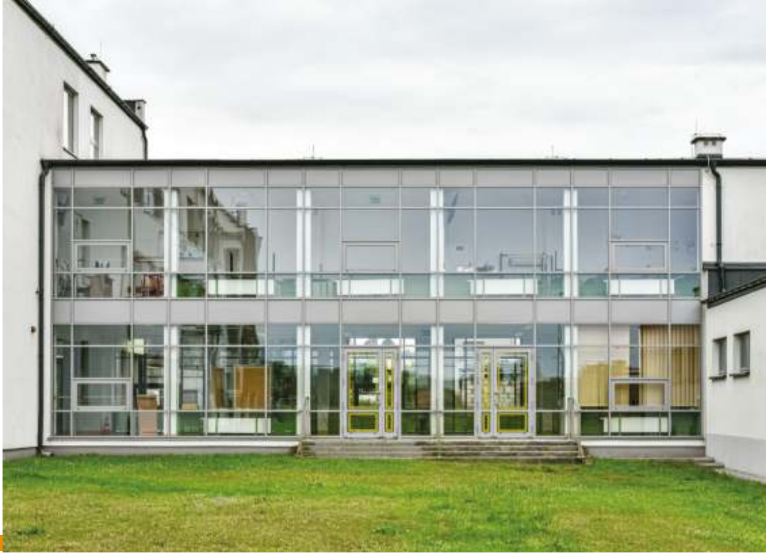
Vocational School Complex, Kurzętnik. 2018
